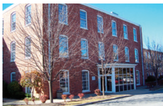
Former Madison Center Building
